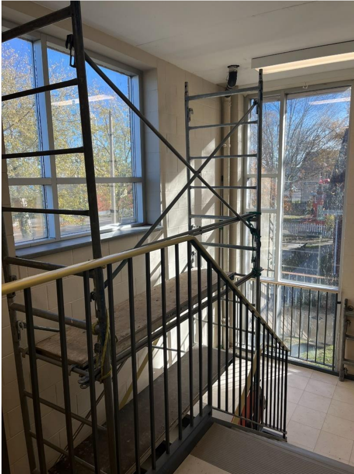
View of east stairwell
