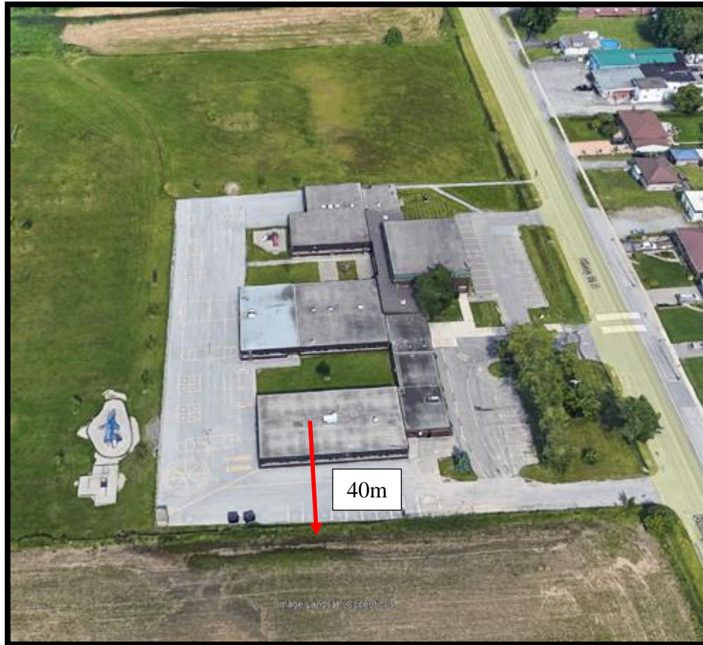
FIGURE 5 ROOFTOP HVAC UNIT TO RECEPTOR LOCATION
