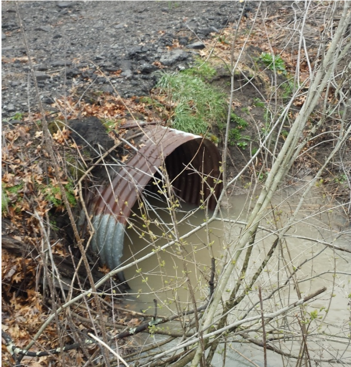
Figure 1: Outlet side of existing 1.2m diameter culvert
