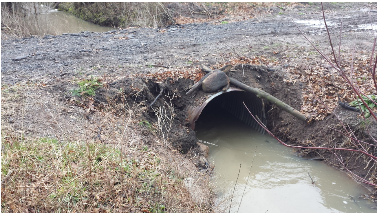
Figure 2: Inlet side of installed 1.2m culvert
