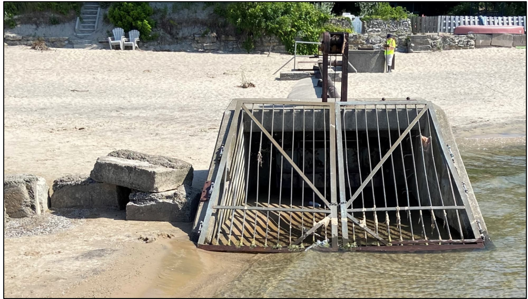
Figure 22 Oil Mill Creek Outlet Structure
