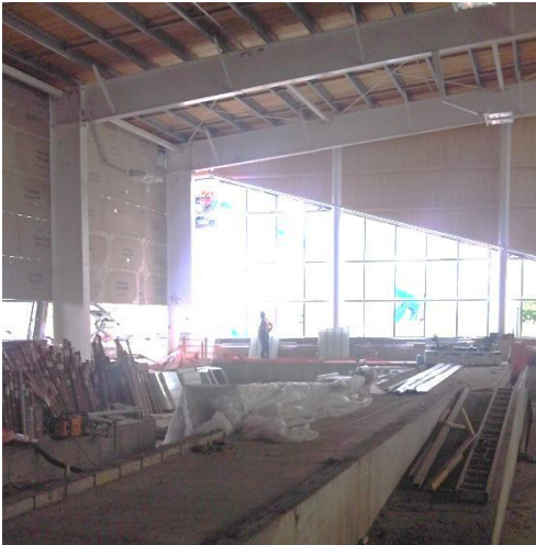
Aquatic centre metal cladding and Kalwall enclosure installation
