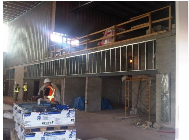
Aquatic change room and administration spaces with YMCA fitness above.
