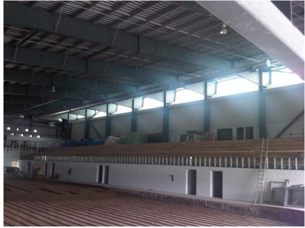
Arena 1 bleacher seats. Rink construction is underway
