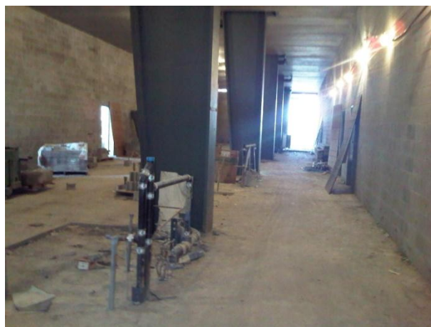
Arena change rooms and corridor - mechanical and electrical installations are ongoing.
