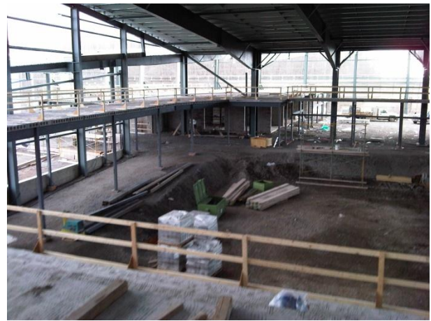
Proposed running track – precast installation is ongoing
