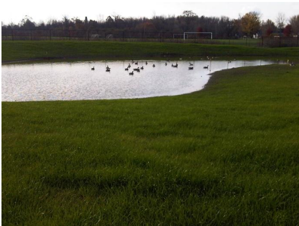
Storm water management pond
