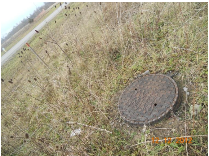
Buried Sanitary Sewer – Adjacent to South site boundary line.
