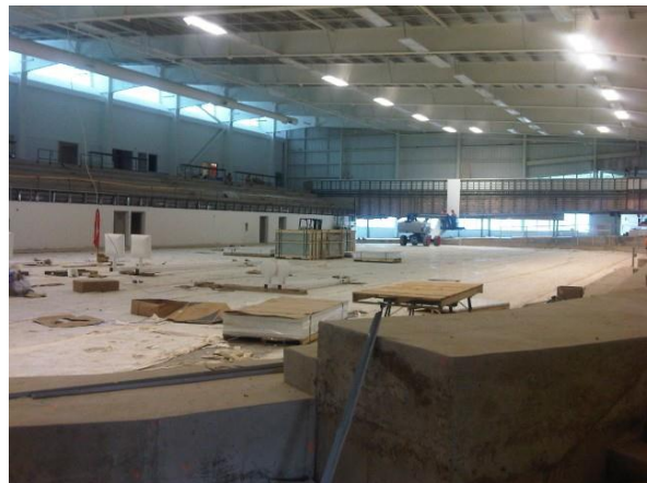
Arena 1 – interior finishes are ongoing.
