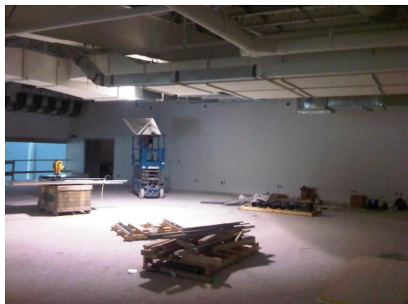
Finish work is underway in the fitness area.
