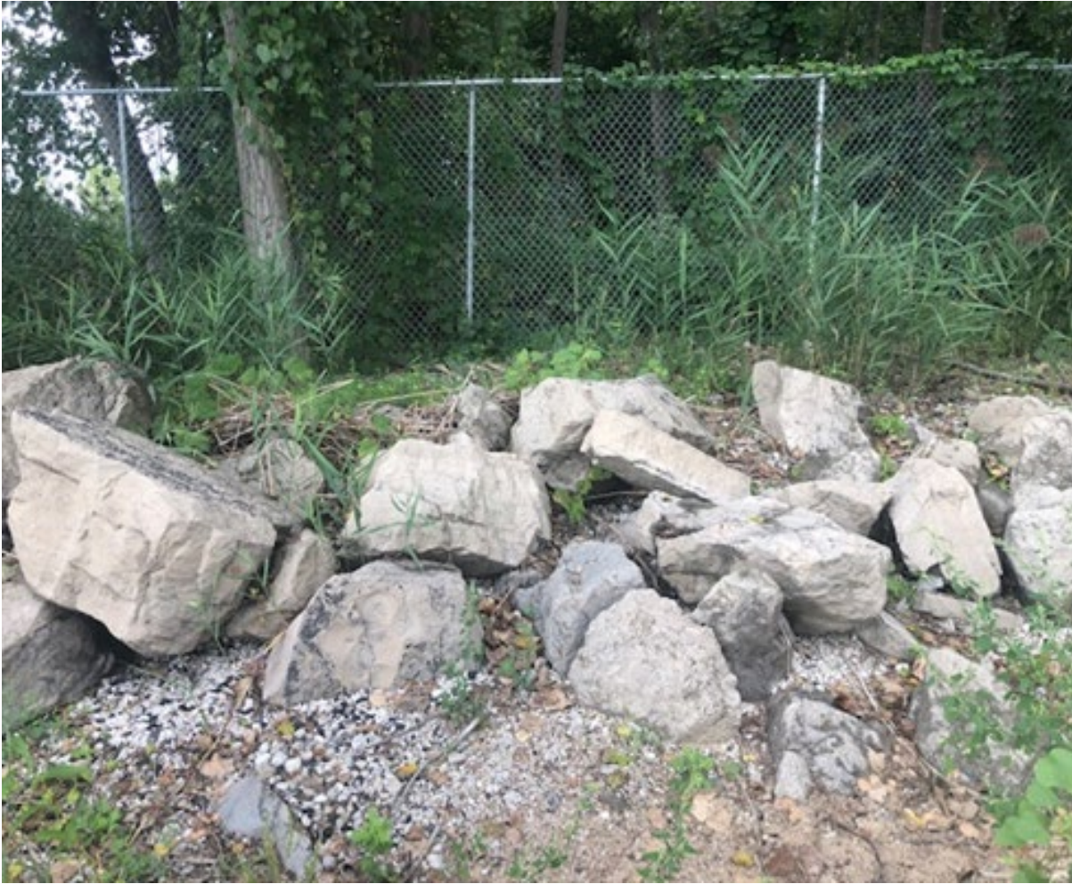
Photograph 3: Rocks and berm at the foundation of the replaced western fence.
