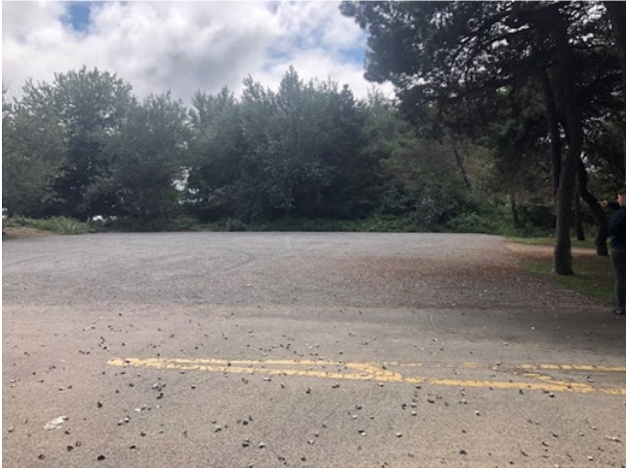
Photograph 5: Gravel area west of entrance access road to be restored with the native bermed material at the western lot perimeter.
