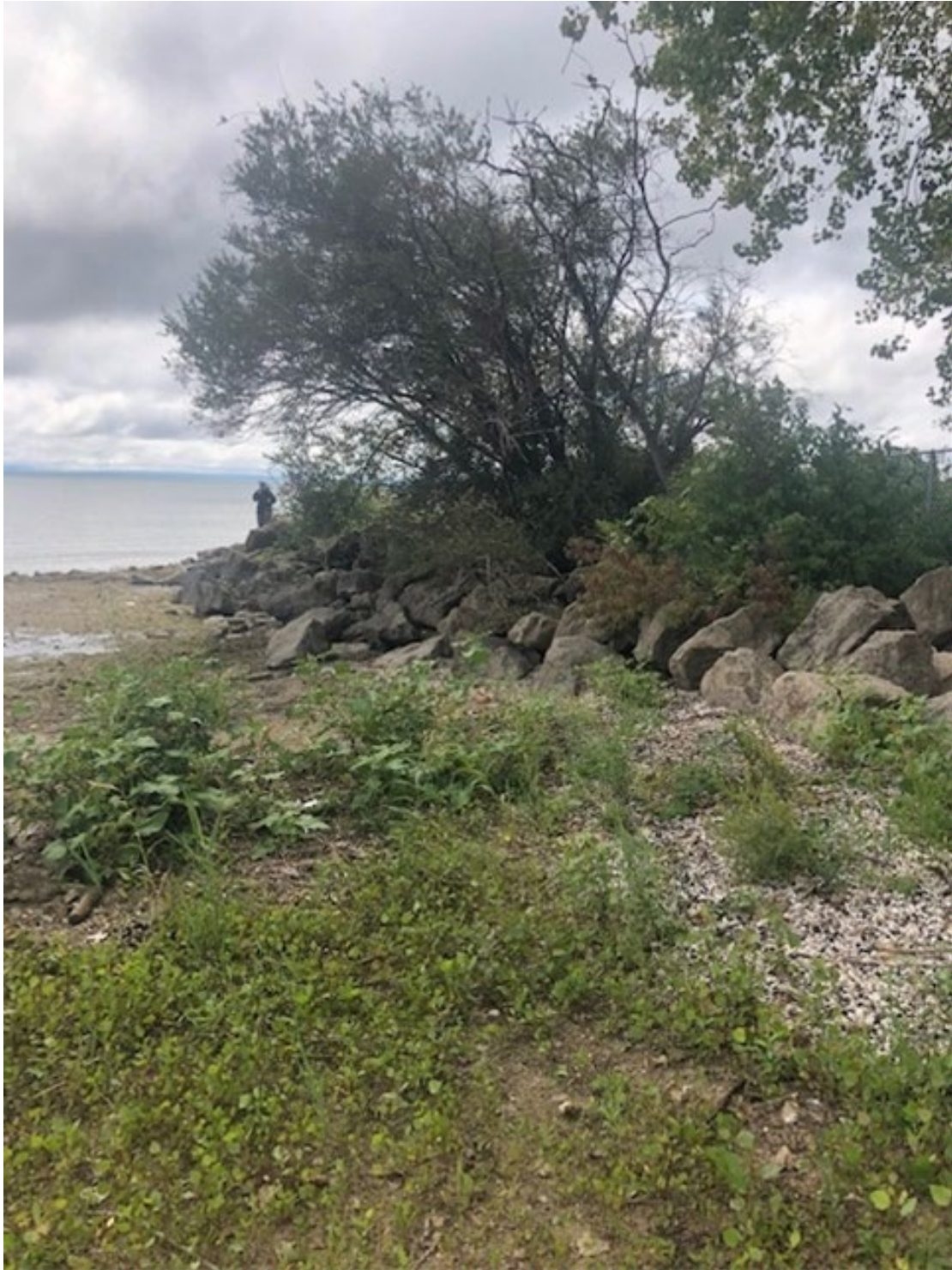
Photo 4: Extent of earthen berm that delineates the western limit of the leased beach area.
