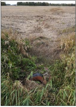
**Figure 4 East Branch Extension looking West** From the photo, it is clear that the existing inlet is not performing well and surface flows are re-establishing along the field.
