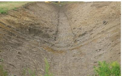
Figure 12 Trapezoidal Ditching Under Construction
