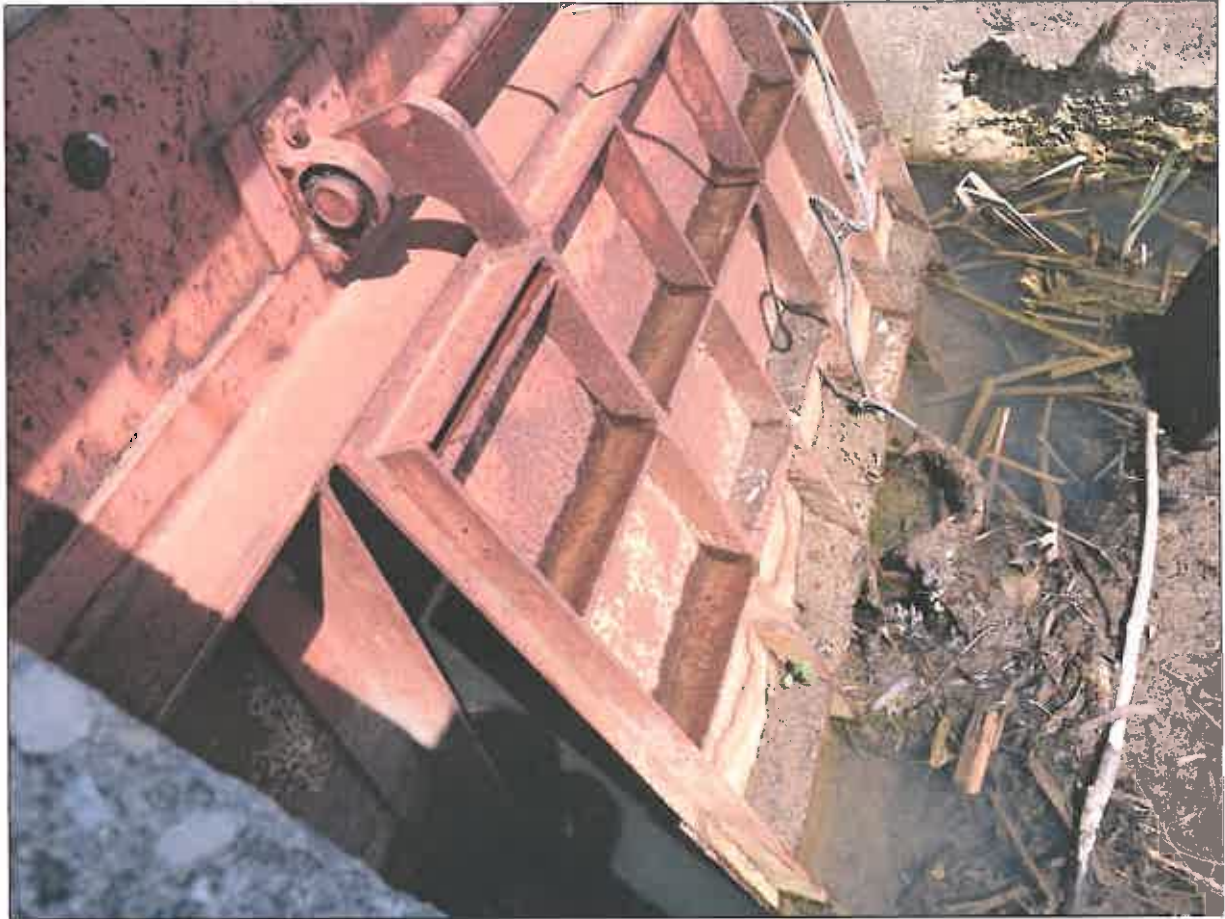
Figure 2-2 Rosemount Ave. Storm Sewer Outlet
